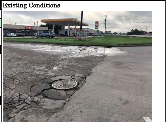
Existing Drainage Conditions at Coronado St.
