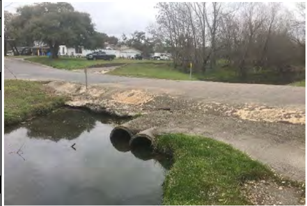
Existing 2 - 24" RCP Culvert (Facing D/S)
