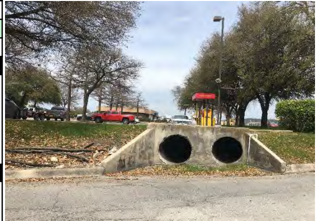
Existing 2 - 36" CMP Culvert (Facing D/S)
