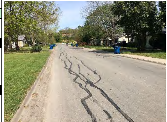
Existing Conditions at Harper Street (Facing U/S)
