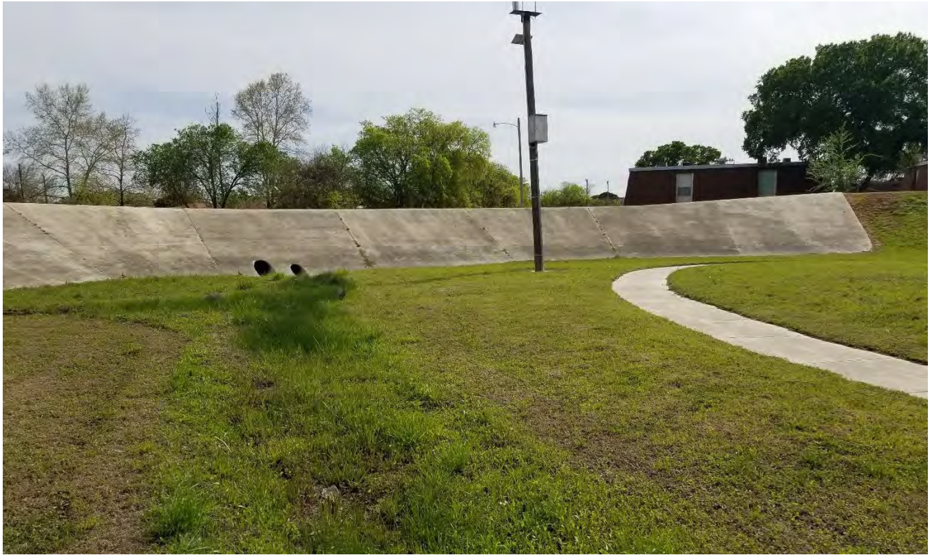
Figure 45 – Outflow Structure for Kroc Center Detention Pond
