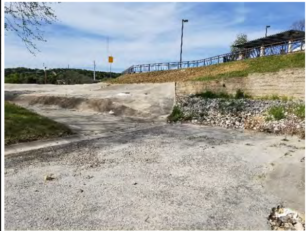
Existing Drainage Spillway - Facing Towards Kroc Center Pond
