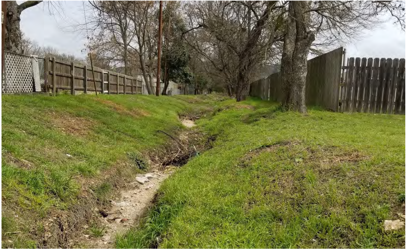
Figure 24 - Earthen Drainage Channel Facing Upstream
